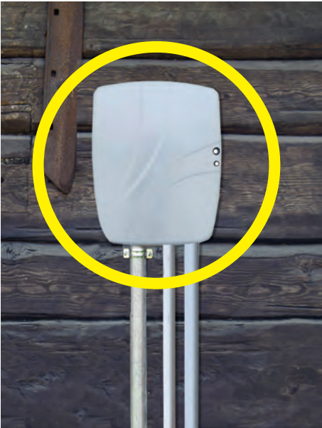
A clamshell must be hung on every home or business to get service.
